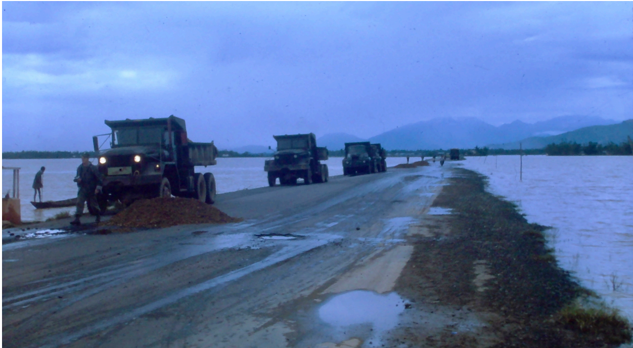
Seabees repairing shoulder on Highway 1, Vietnam 1970-71
